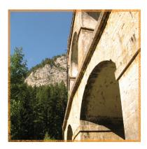
The Semmering railway line, which was planned and built by Carl Ritter von Ghega, was completed in 1854. Across an overall track length of 41 km the Semmering railway overcomes an altitude difference of 460 m and passes 15 tunnels and 16 viaducts. Due to the harmonious blend of nature and technology and the unique construction technique of the railway it was declared a UNESCO World Heritage site in
